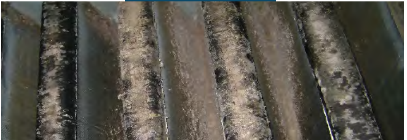
Contaminated AC coils
